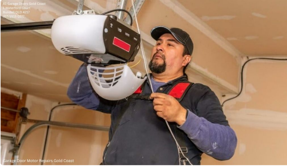
Garage Door Motor Repairs Gold Coast
